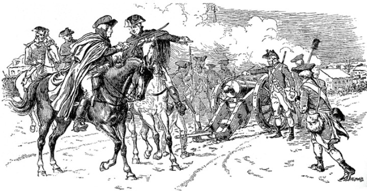
Second Crossing of the Delaware December 30, 1776
